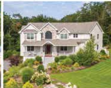
Essex Custom Built 32 River Road Drive Builder's Home Offered at $1,895,000
