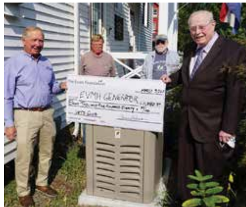
The Essex Foundation President Bruce Glowac (front left) presents a ceremonious check to Essex Veterans Memorial Hall President Art Davies as fellow House Committee members Tim Comstock (back left) and John Pianta stand behind the new standby generator.
